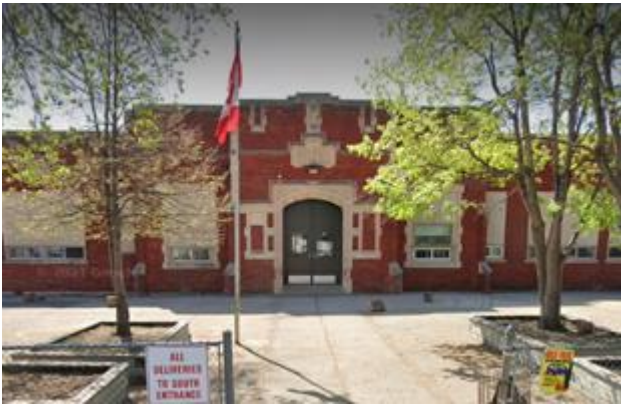
Windsor School – 80 Cunnington Ave; Grades 1-9
